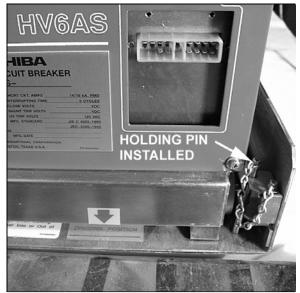
Fig. 20 Breaker at DISCONNECTED Position
